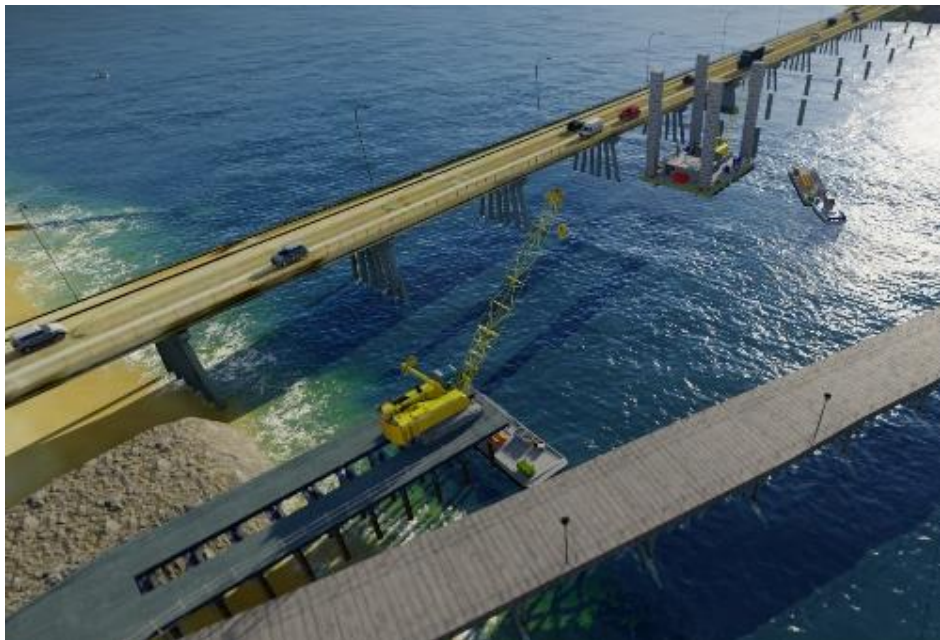
Artist impression of the temporary wharf and jack up barge in operation
